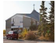
Valleyview Community Church
