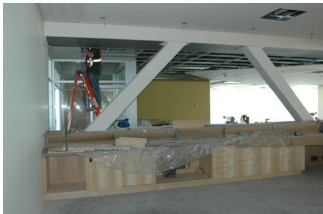
new shelving for the main reception area
