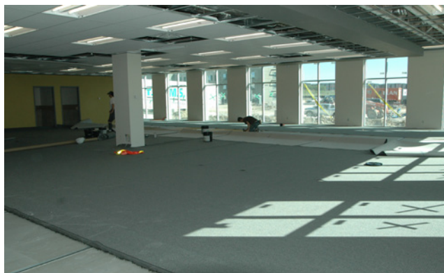
new carpeting is installed in the Ambrose Library
